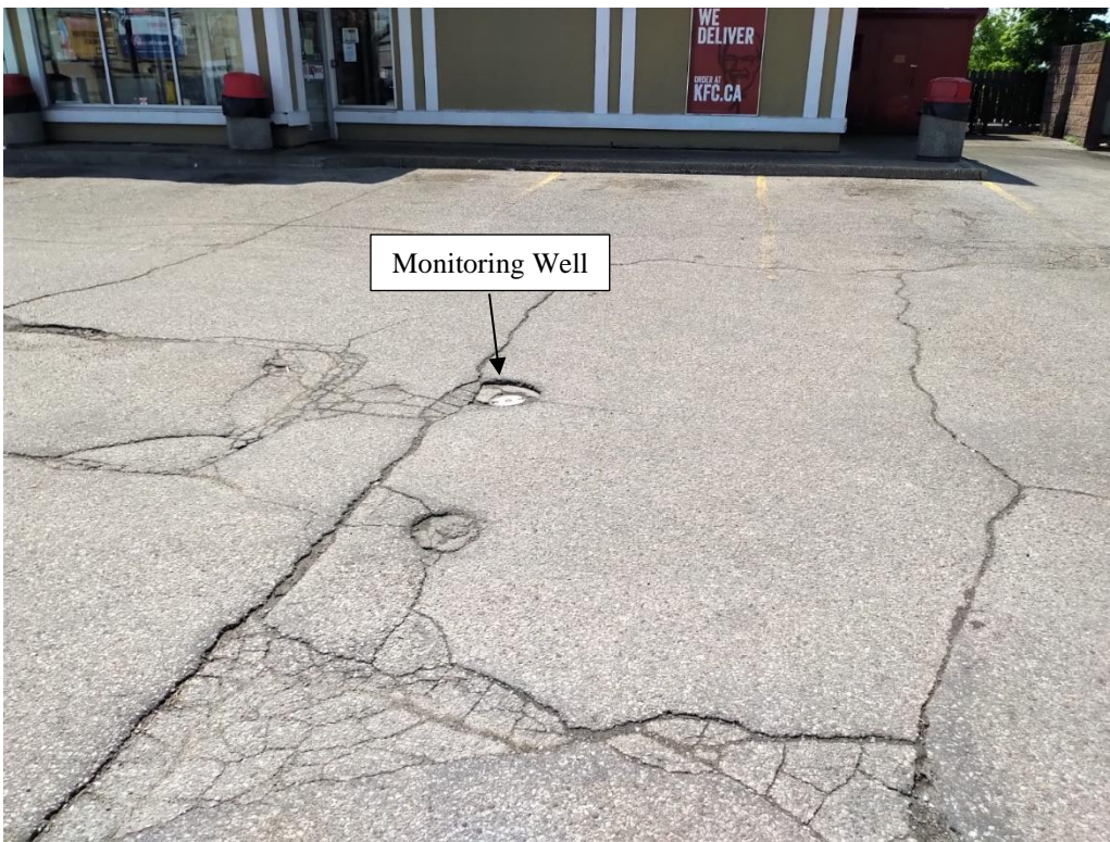
Photograph No. 12 – South facing view of Kentucky Fried Chicken located at 27 Colborne Street East, which included a monitoring well.
