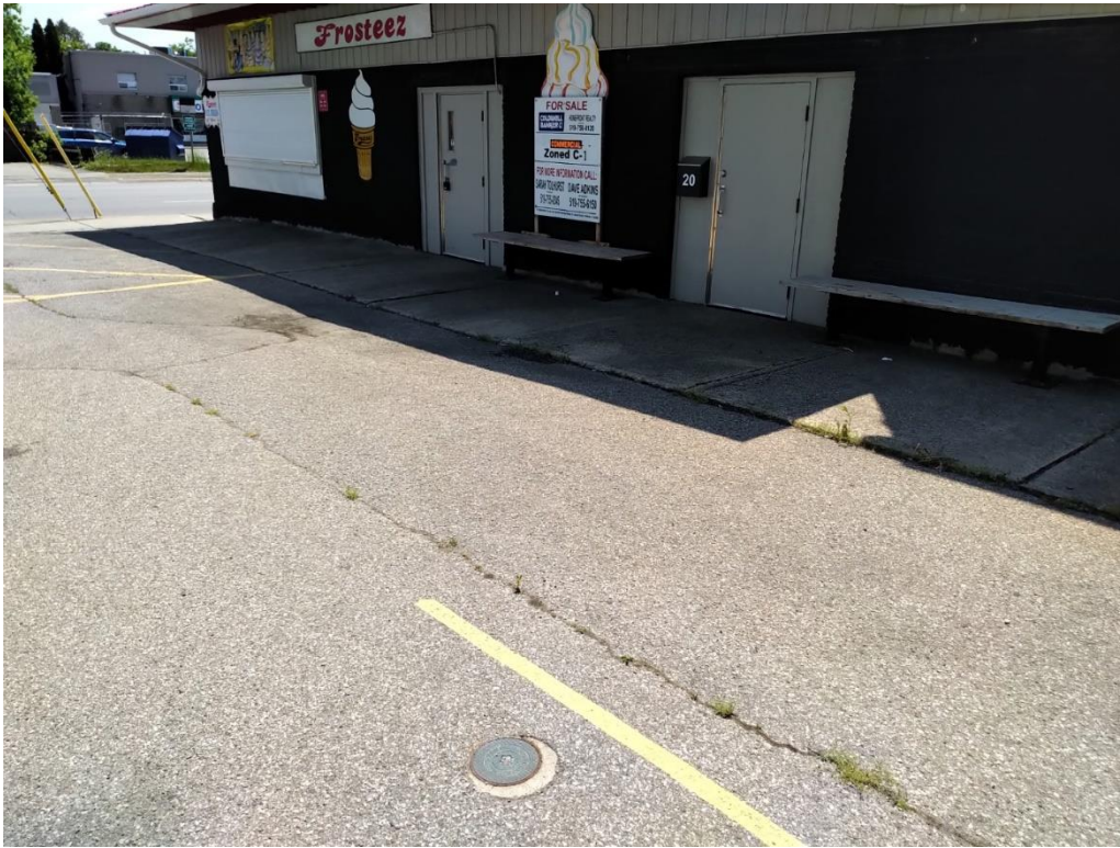
Photograph No. 3 – Southeast facing view of 20 Clarence Street, depicting a monitoring well.
